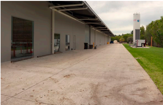
Geothermal Loops installed below nature strip
